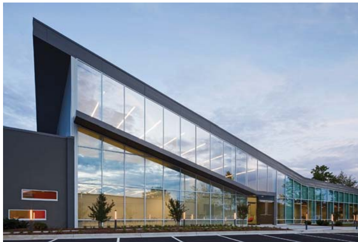
Transurban Operations Center Credit: Ron Blunt
